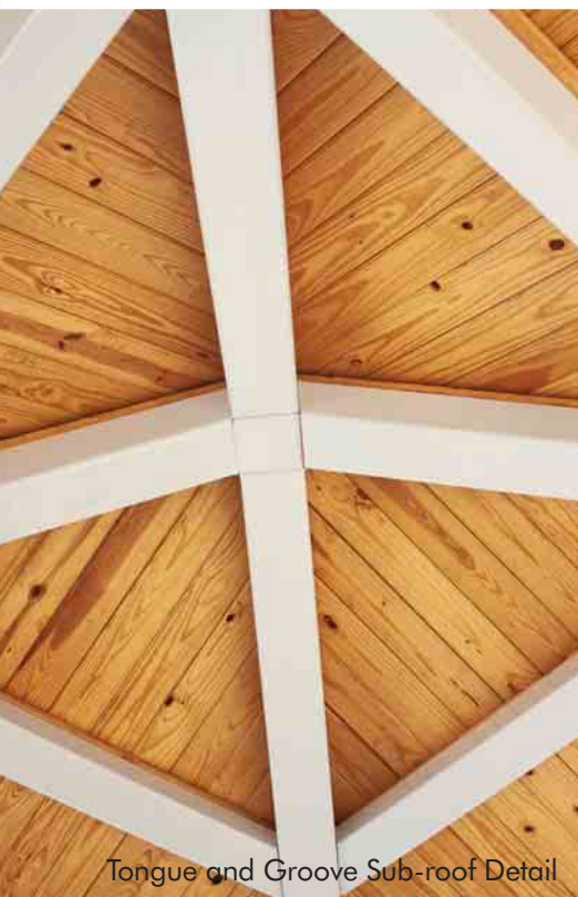
Tongue and Groove Sub-roof Detail
